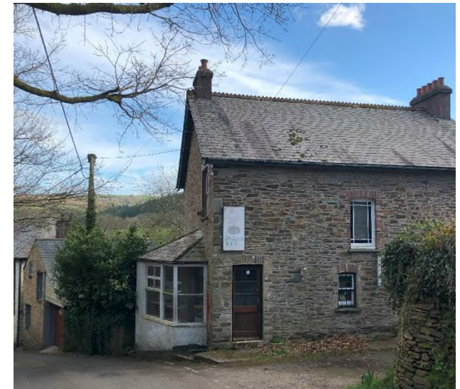
Photo alongside: The former Village Stores, Luckett
